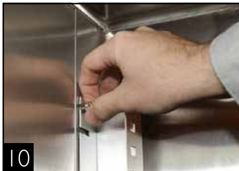
Pilaster installation (side wall of cabinet)
