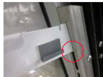
Bottom notch installed (no gap)
