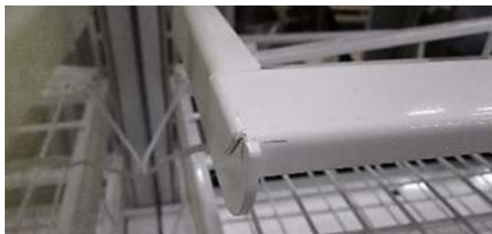
Light assembly installed on shelf support
