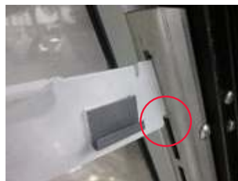
Top notch installed (gap)
