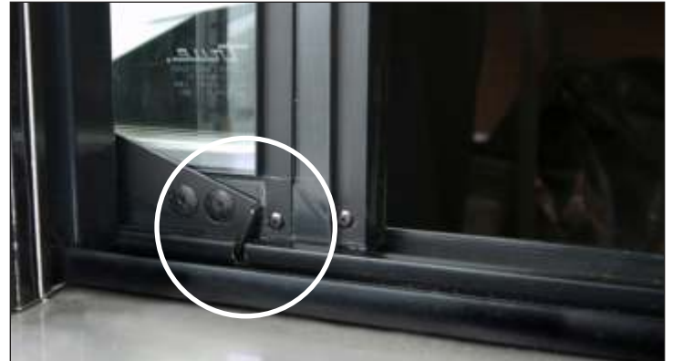
Fig. 1. Door latch is in the open position (engaged with notch).
