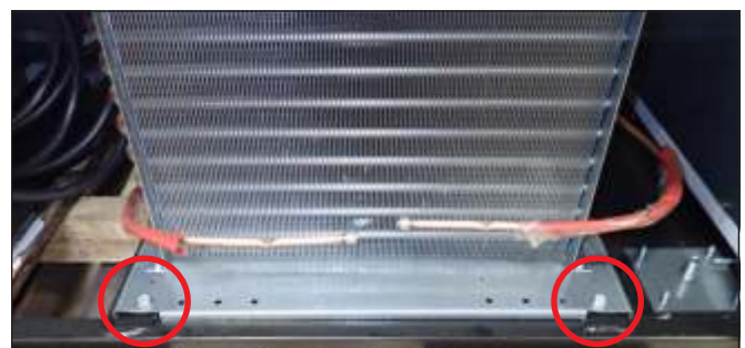
Fig.4. Remove condenser base bolts.
