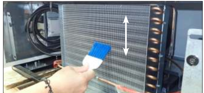
Fig. 2. Never brush across the coil fins.
