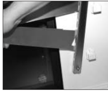
Fig. 6. Hook the shelf supports into the pilasters at the desired height.
