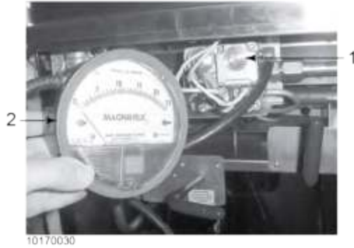
Figure 2-15 Adjusting Regulator
