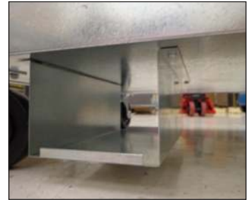
Fig. 3. Secure the HDP bracket to the underside of the cabinet.
