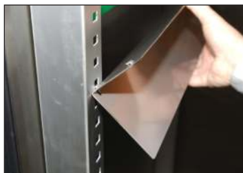
Fig. 7c. Installing kit #3 universal tray sides.
