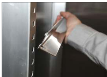
Fig. 7a. Installing kit #1 angle tray sides.
