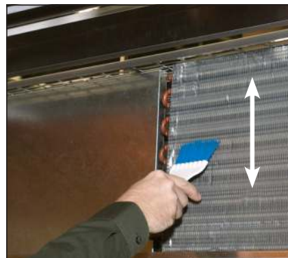
Fig. 3. Never brush across coil fins.
