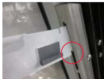
Top notch installed (gap)
