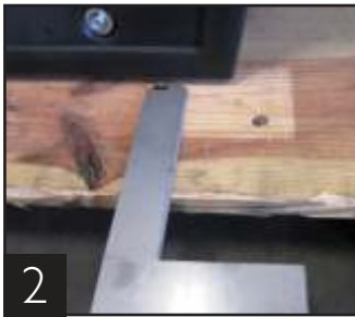
Removing bracket from cabinet.
