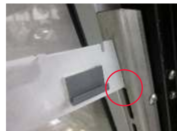
Bottom notch installed (no gap)
