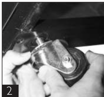
Thread castors into existing leg leveler holes.
