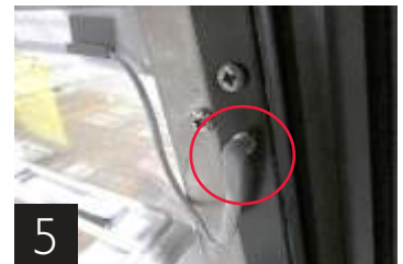
Light cord installed
